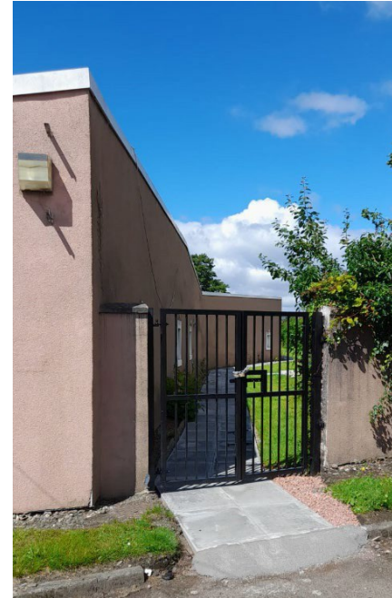
Completed new gate at Willox Park
