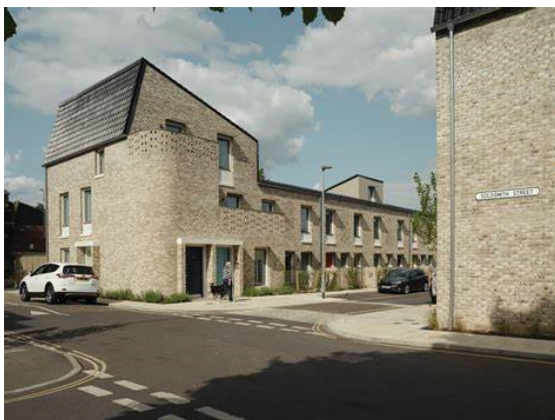
Goldsmith Street, Norwich is a development of ultra-low-energy homes which are estimated to reduce annual energy costs for residents by 70%.
