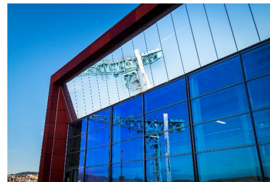
The Queens Quay Energy Centre. Clydebank supports an energy network for the whole Queens Quay site with network connections available for sites to the north of Glasgow Road. The iconic design of the building makes it landmark at the waterfront to complement the Titan Crane.
