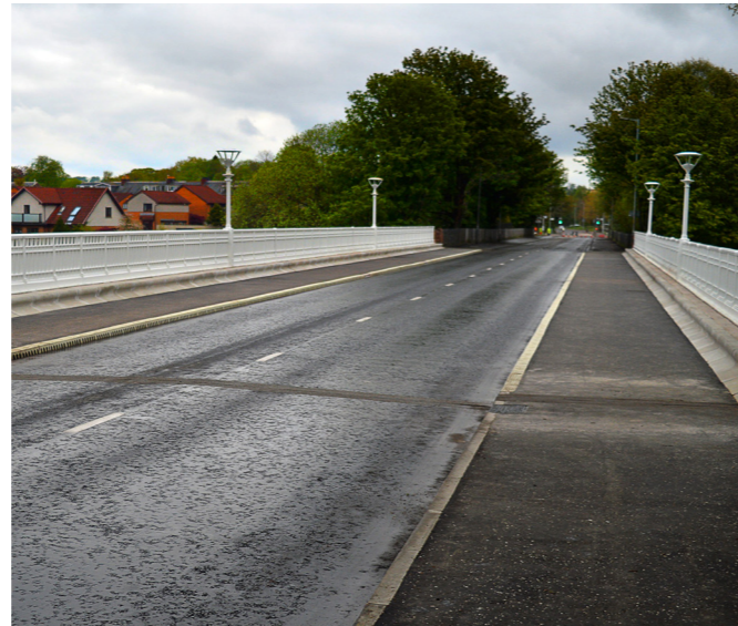
Completed the £3.6 million restoration and refurbishment of Lomond Bridge as part of significant regeneration works in Balloch
