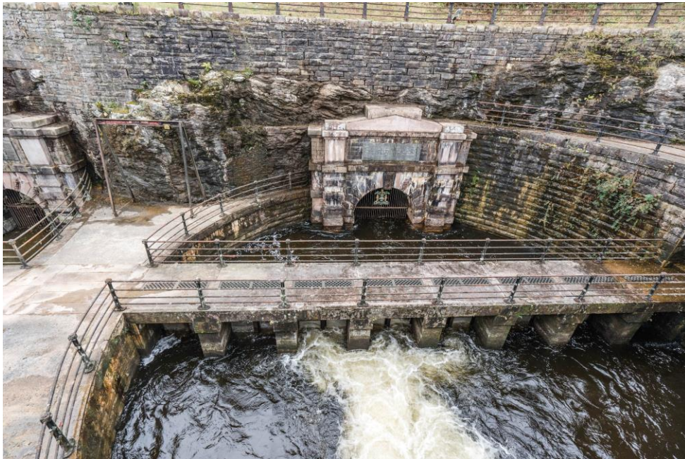
Loch Katrine Water supply Aquaducts
