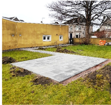
New outdoor patio area at Willox Park for garden parties etc.
