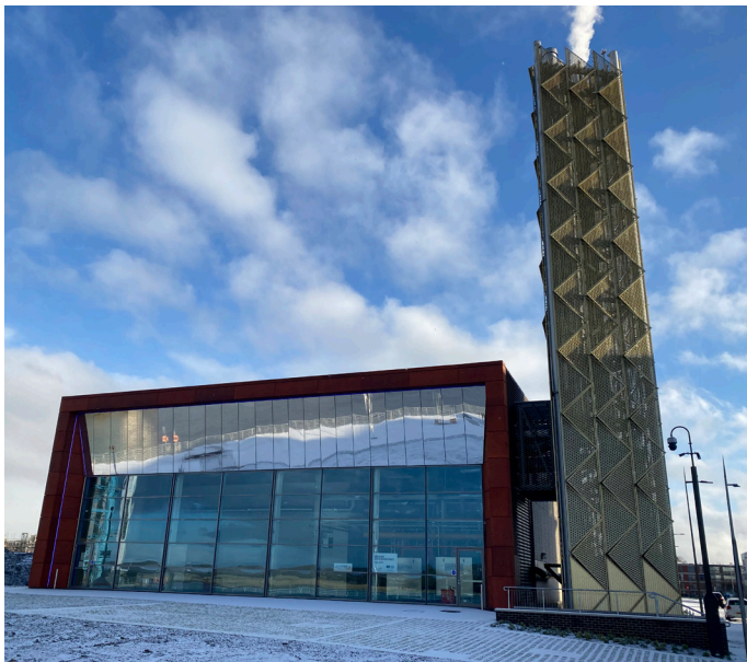
Launched Queens Quay Energy Centre
