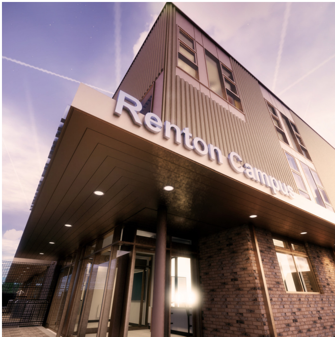
Progressed construction at Renton Campus
