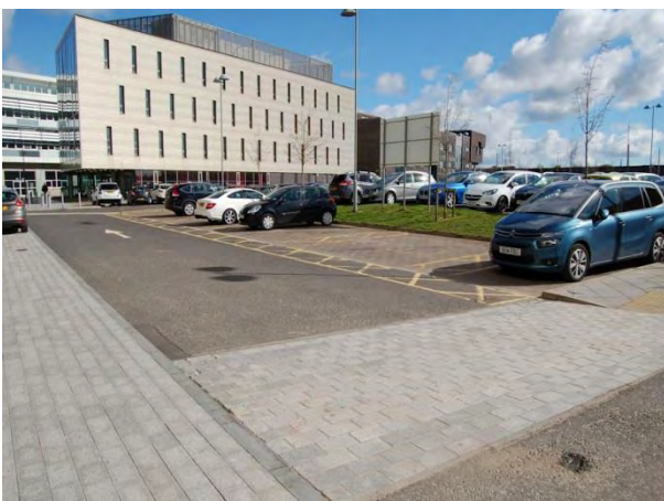
Disabled Parking Bays
