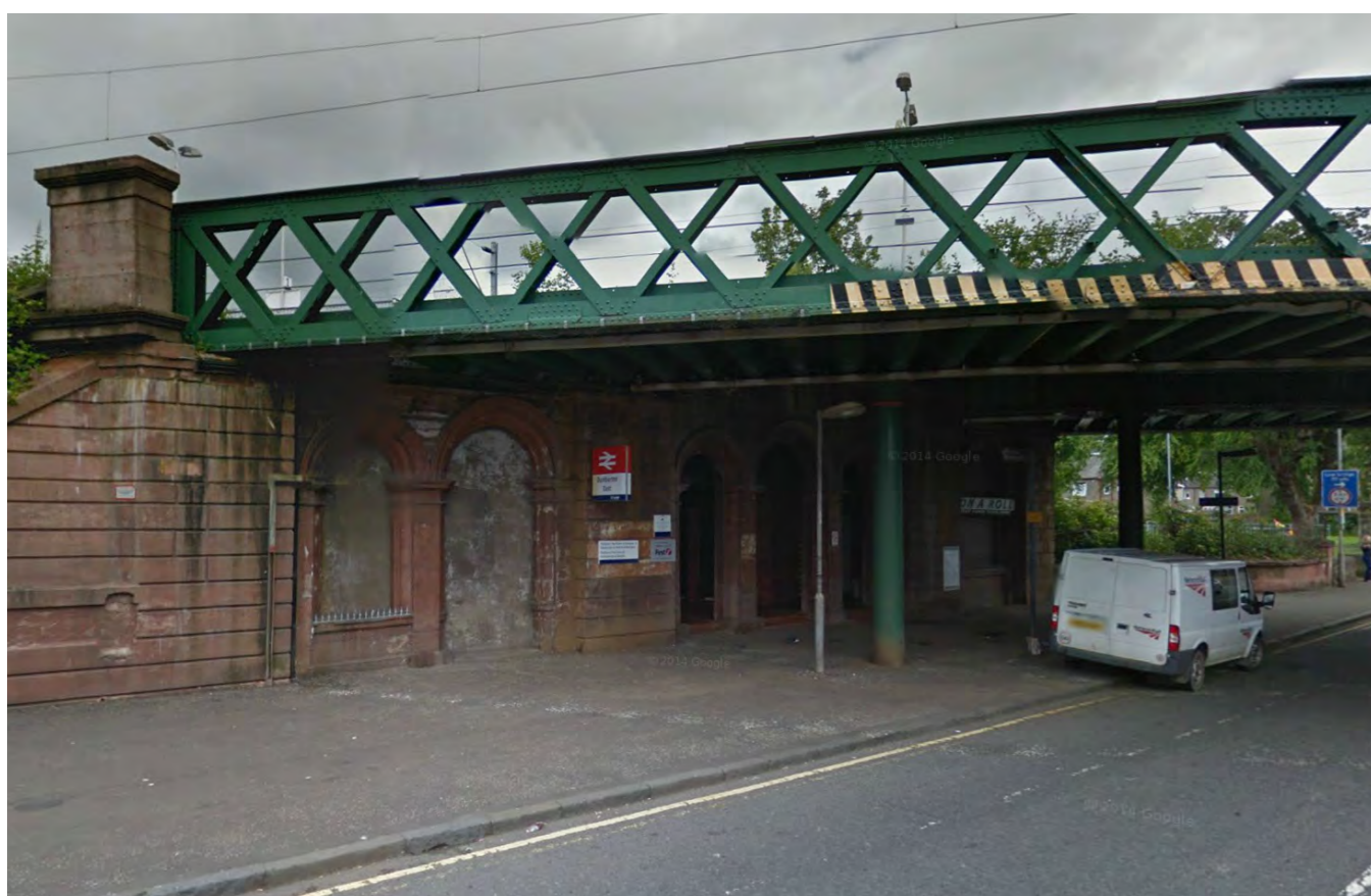
Dumbarton East Station Entrance
