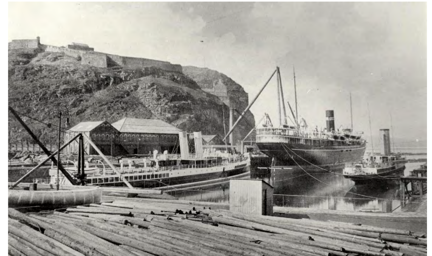
17. New dock at Leven Shipyards at the foot of Castle rock from the north c1906 (courtesy of West Dumbarton Libraries & Cultural Services)
